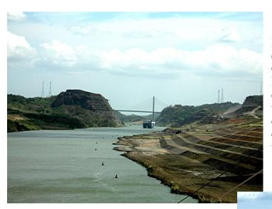
Here is a photo of the Gaillard Cut (formerly known as Calebra Cut) with Gold Hill on the left and Centennial Bridge for the Pan American Highway over the Canal in the background. The terraced hillside on the right is a result of the constant effort to control erosion of dirt and rock into the Canal and also to widen the narrow places.
