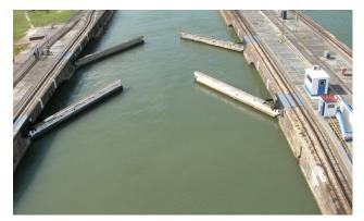
After the lock was filled with water and the ship raised to the next level the gates were opened so we could proceed.
